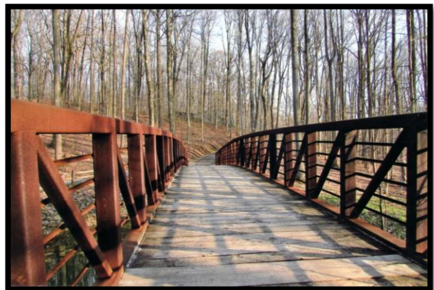
May 2nd: WV Wildlife Center Bridge – Linda Perrine
